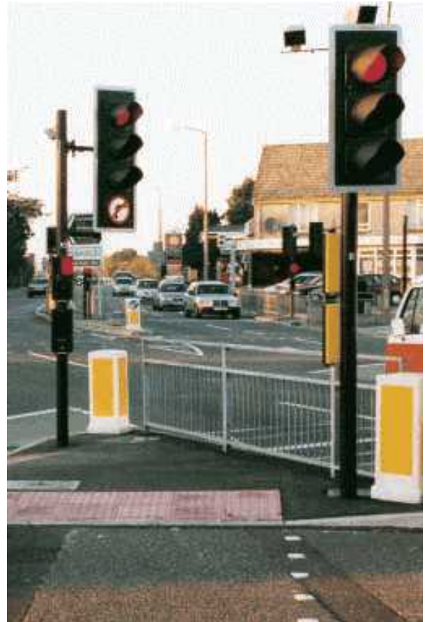
Near side facility at a junction
