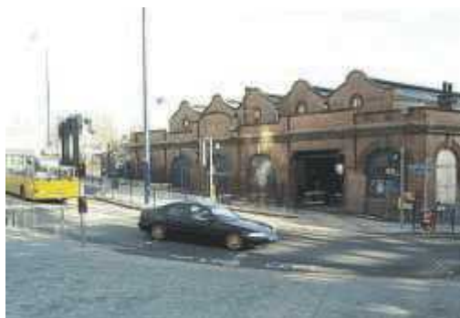
An example of a wide crossing
