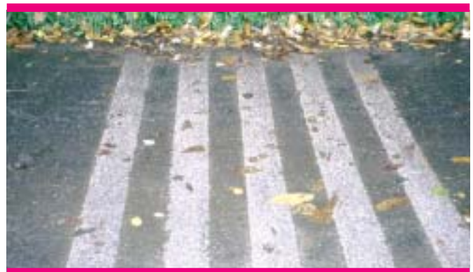
False Cattle Grid, Comp Lane in Kent
