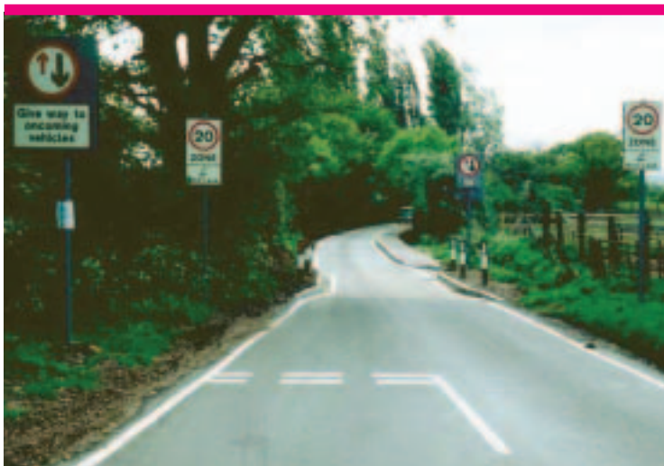
Northern entry to the scheme (left) had a greater speed reducing effect than the southern gateway
