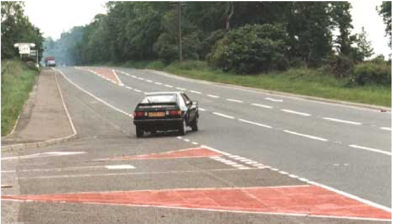
Plate 6 Coloured Surfacing used to Improve Contrast in the Island Area of Priority Junction
