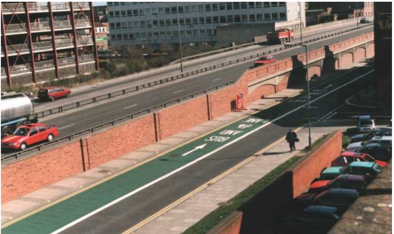
Plate 7 Coloured Surfacing used to Supplement Road Markings on a “Contraflow” Bus and Cycle Lane
