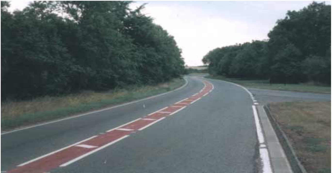
Plate 3 Coloured Surfacing used to Improve Contrast Along Sections of Sub-Standard Visibility
