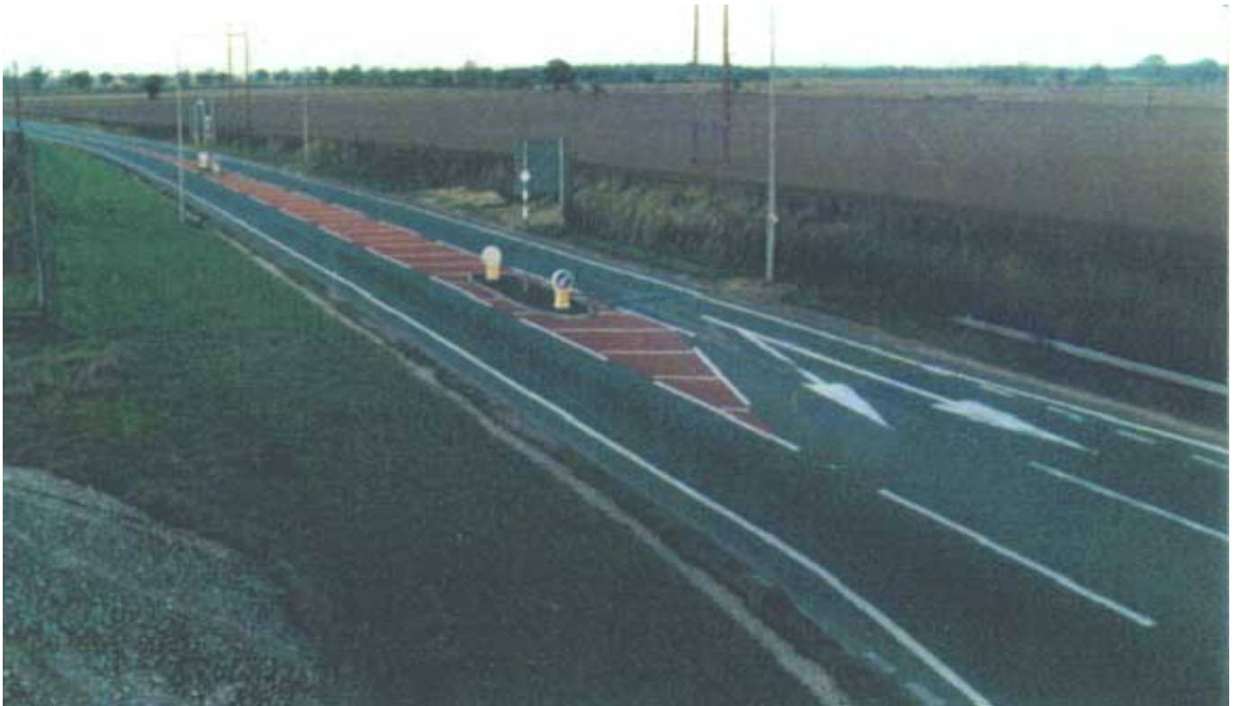
Plate 2 Coloured Surfacing used to Improve Contrast on a Mainline Junction Approach
