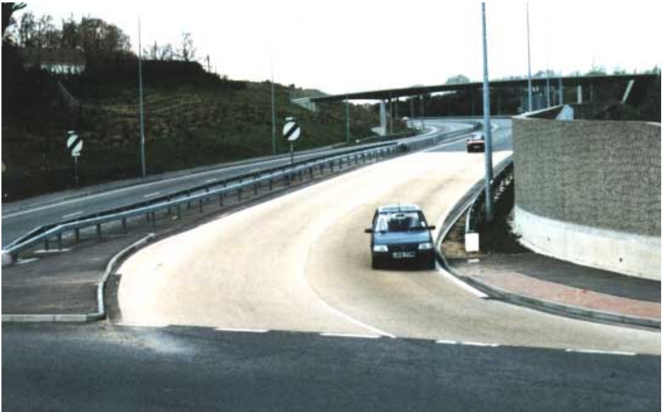
Plate 10 Coloured Surfacing highlighting a change in the road layout, a by-product of High Skid Resistance Surfacing applied at a junction to reduce the risk of skidding.
