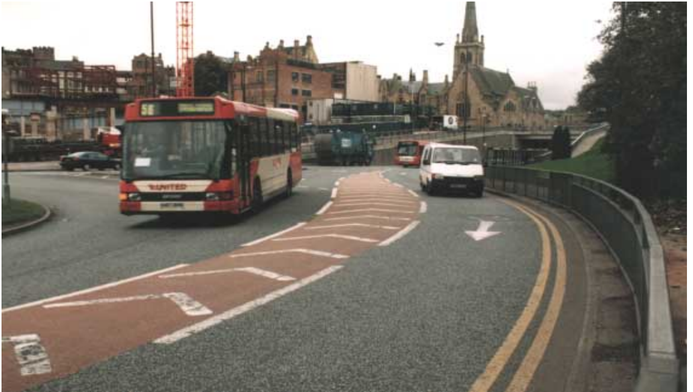
Plate 5 Coloured Surfacing used to Improve Contrast on a Segregated Left Turn Lane at a Roundabout
