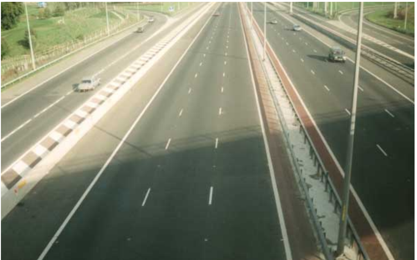
Plate 4 Coloured Surfacing used to Improve Contrast Along Margins to Deter Over-Running
