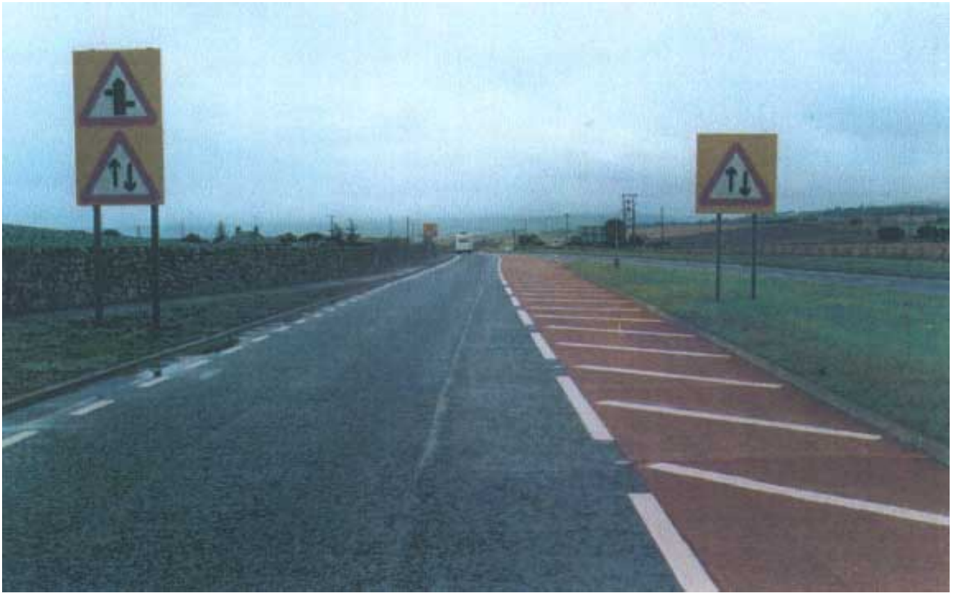
Plate 1 Coloured Surfacing used to Improve Contrast at Change in Cross Section (Dual to Single)
