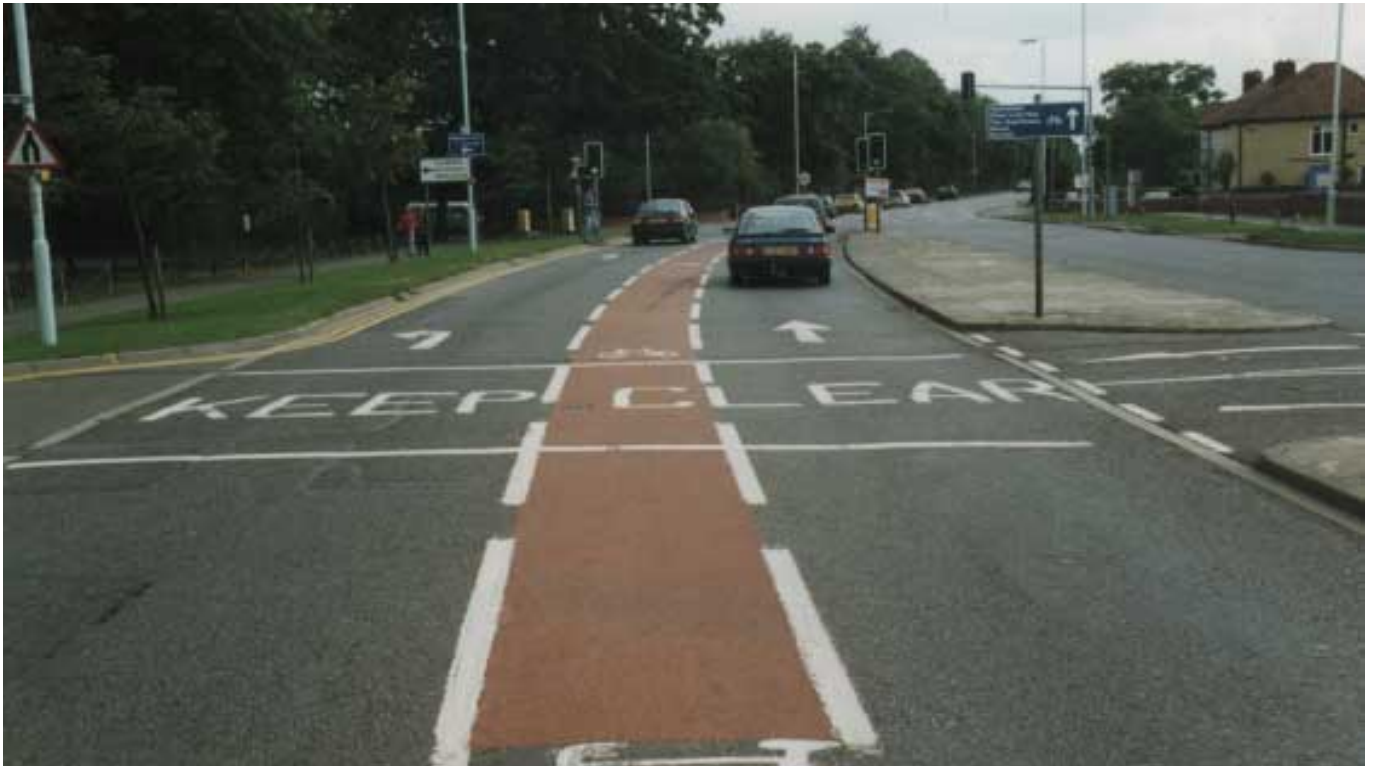
Plate 9 Coloured Surfacing used to Supplement Road Markings for a Cycle Lane
