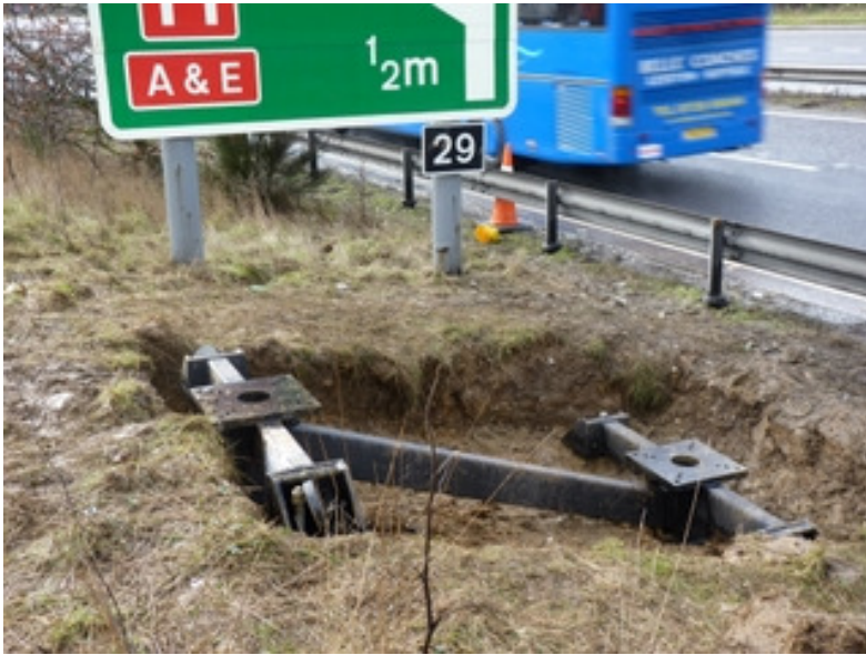
H Frame installed on site at the A12.
